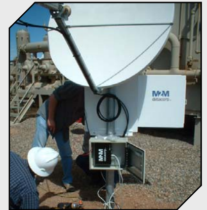
VSATs (very small aperture terminals) provide satellite connectivity from compressors to the M2M’s data center in Denver, Colorado.
